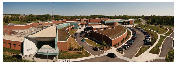
Saint Elizabeths' Green Roof
